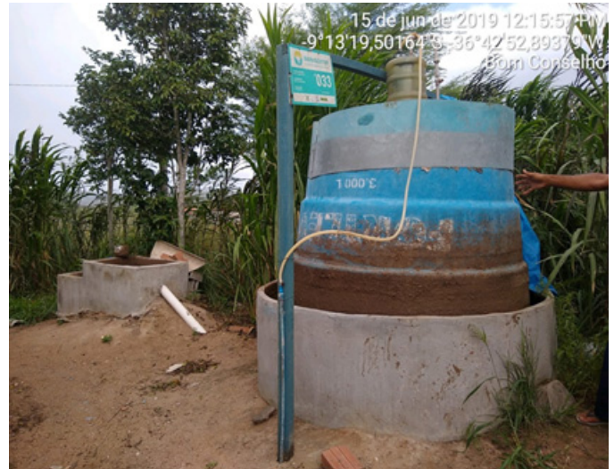
Figure 2 – Sertanejo biodigestor with maximum biogas load. Angico Site, Bom Conselho-PE, by Wanderley Nunes and Cláudio Almeida, 2020.
