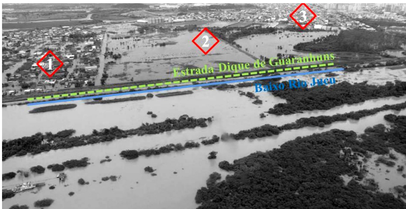
Figure 7 – Flooded neighborhoods after the December 2013 rains, Espírito Santo, Brazil.
