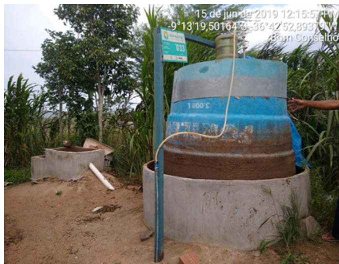
Figure 2 – Sertanejo biodigester with maximum biogas load. Angico Site, Bom Conselho-PE, by Wanderley Nunes and Cláudio Almeida, 2020.
