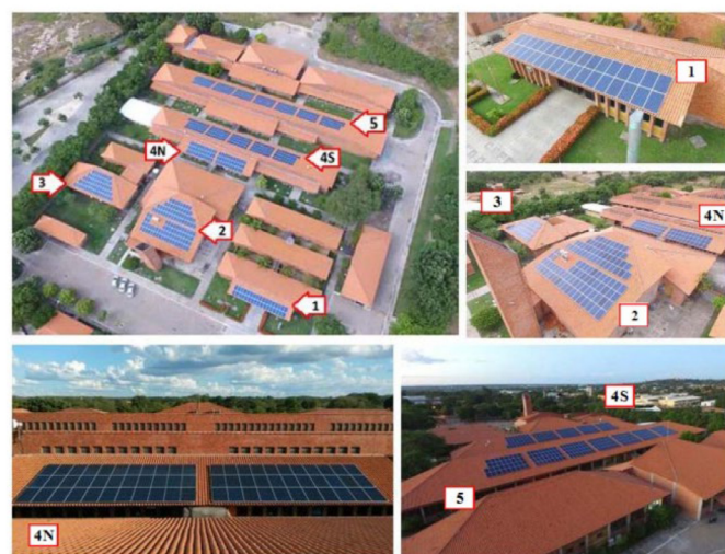
Figure 3 – Detailed view of the GCPVS installed at IFPI's Floriano Campus. Source: Morais et al. (2019).
